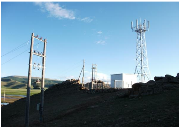
Unitel 20 m Tower, 4x4 shelter, 10/0,4kV Power System, Arkhangai Province
