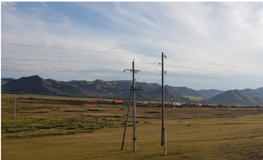
10/0.4kV transmission line
